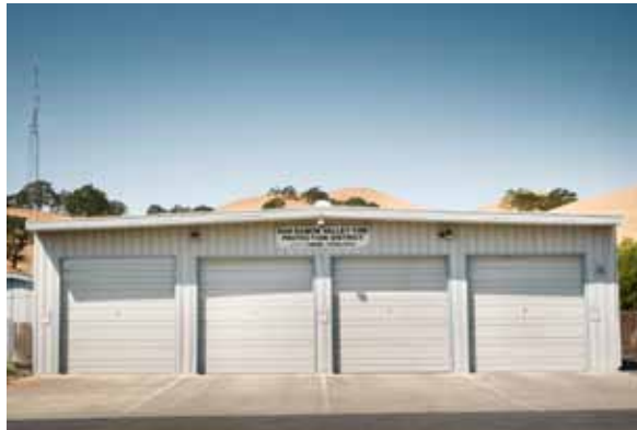
Training 6100 Camino Tassajara Road Tassajara
